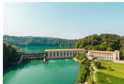
Mühleberg Capacity: 45.0 MW End of the concession: 2097
