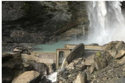
Schattenhalb 1 Capacity: 2.3 MW End of the concession: 2097
