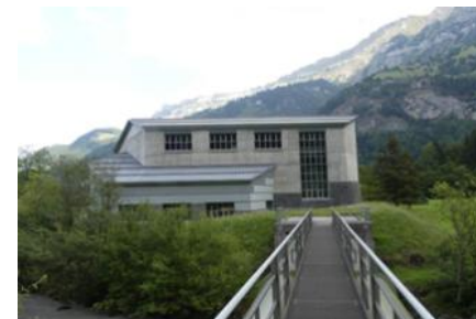
Kandergrund Capacity: 18.8 MW End of the concession: 2071
