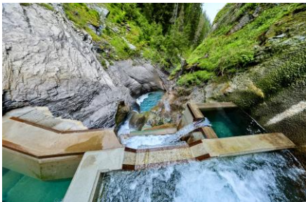
Kraftwerk Sousbach AG Capacity: 11.3 MW End of the concession: not yet determined
