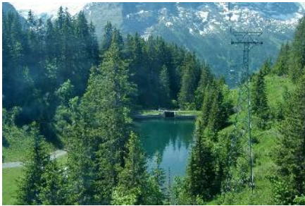
Isch Capacity: 1.5 MW End of the concession: 2041
