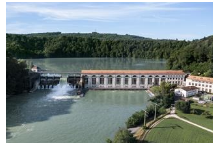
Mühleberg Capacity: 45.0 MW End of the concession: 2097
