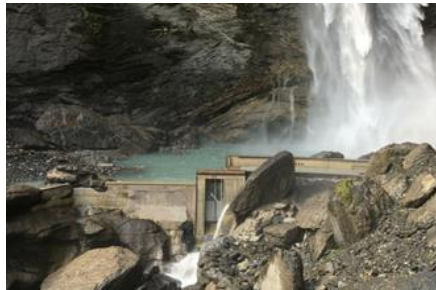
Schattenhalb 1 Capacity: 2.3 MW End of the concession: 2097
