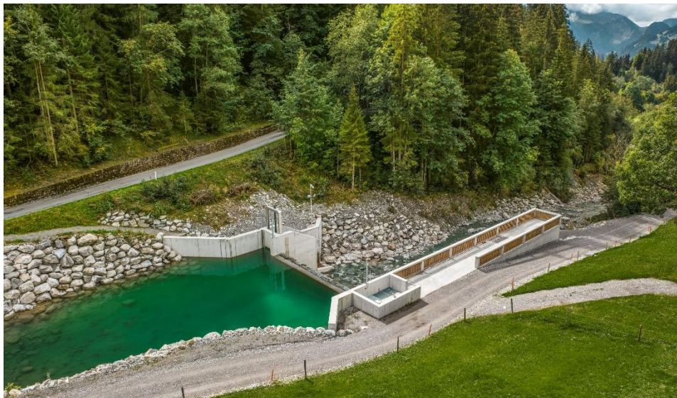
The water catchment at the Turbach hydropower plant © BKW
