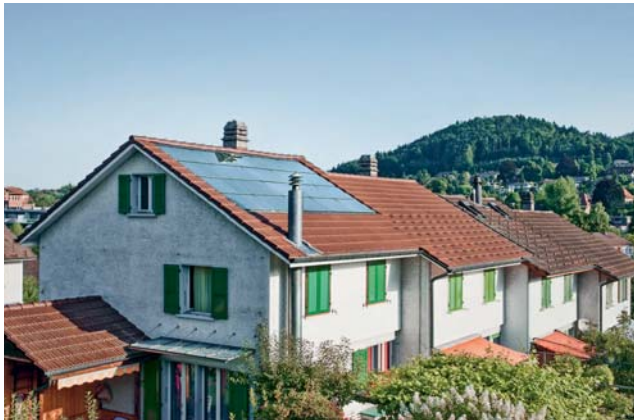
■ Distributed generation from solar power for local use.
