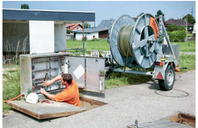
■ An electrician connects cables to the grid.
