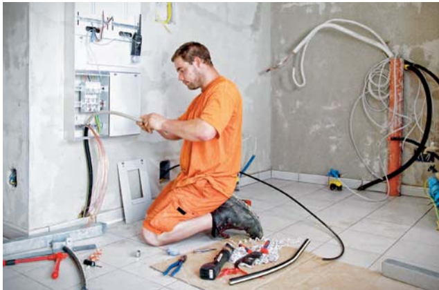
■ An electrician installs cables and wiring in the home.
